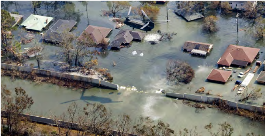
In the middle of this picture you can see the break in the levee.
